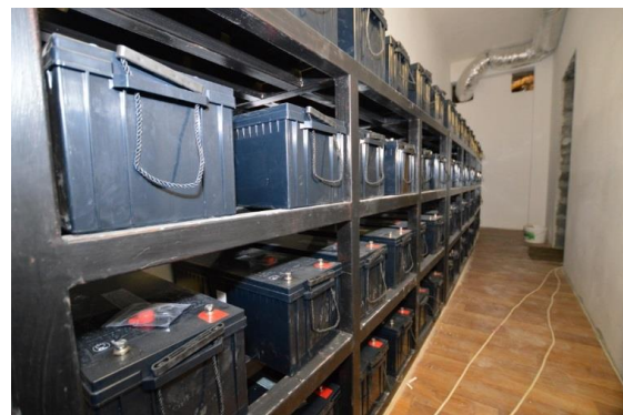
5 Custom Battery Rack Fabricated on Site
