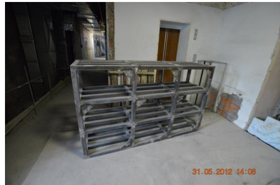
5 Custom Battery Rack Fabricated on Site
