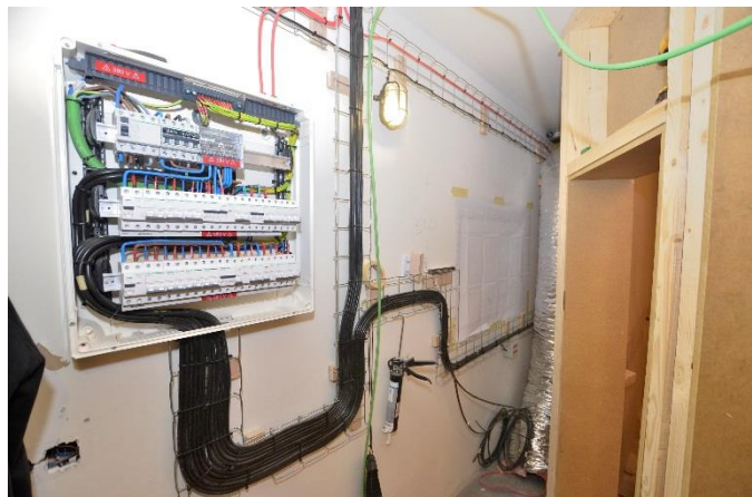
6. A local sub-distribution board in a recording studio service area under construction providing a local radial topography that will match the audio installation layout. (Barcelona)
