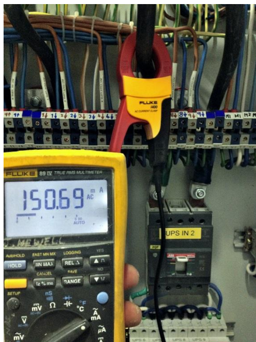
9. Testing system max current load on half of the audio system during commissioning. (150A)
