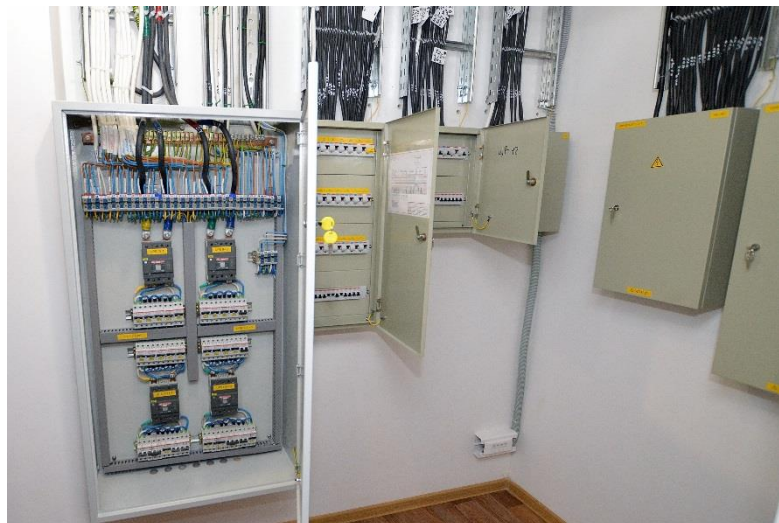
3. 500A (2 x 250A) Audio / Video systems only power room for a film post production studio (CP Productions / NTV Kino – Moscow)
