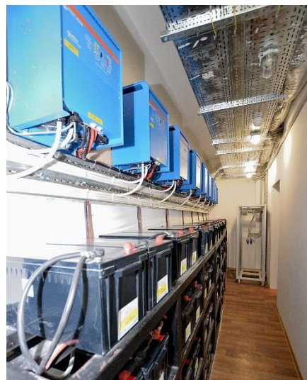
8. - 90KW (180KW peak) of off-grid power units providing a hard-bypassed central single phase backup inverter solution for an entire film post-production facility. - No I.T. UPS could cope with this. - System comprised of Nine Victron Energy Quattro 10KW Marine power units parallel linked in two banks in seamless switch-over UPS mode. 12 hrs backup capacity - (Moscow)
