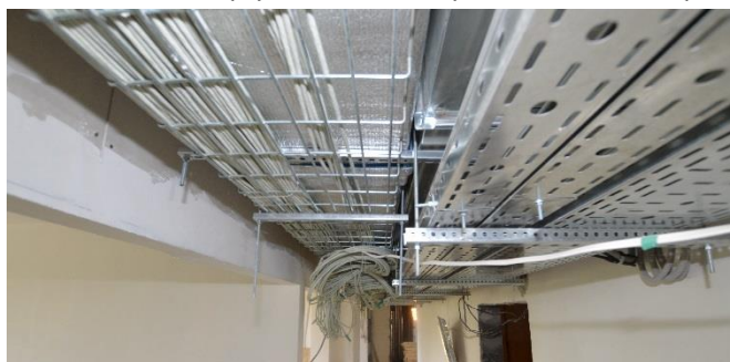
5 All technical service cables in a film post production complex following a common route with minor segregation distances to avoid creating a loop in the ground conductors.
