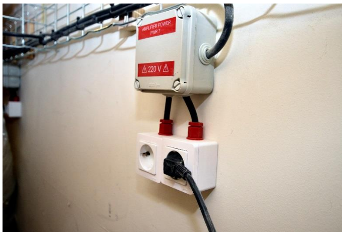
7. A 6mm cable fed from 16A breaker supplying two European 16A power outlets for the audio amplifiers in a recording studio. A terminal box is required to terminate the 6mm cable into the domestic sockets via 2.5mm short links.
