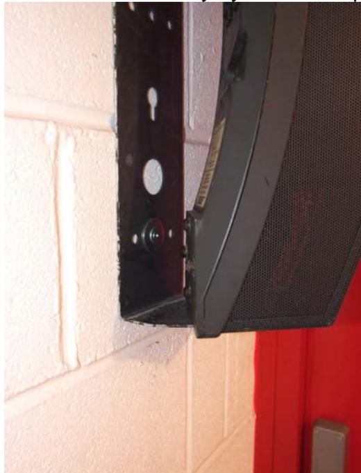
Loudspeaker two was fixed to the structure by means of a piece of unistrut in which was bolted two isolation mounts of the type used by the UK's leading night club chain. The bracket was then bolted to this assembly.
